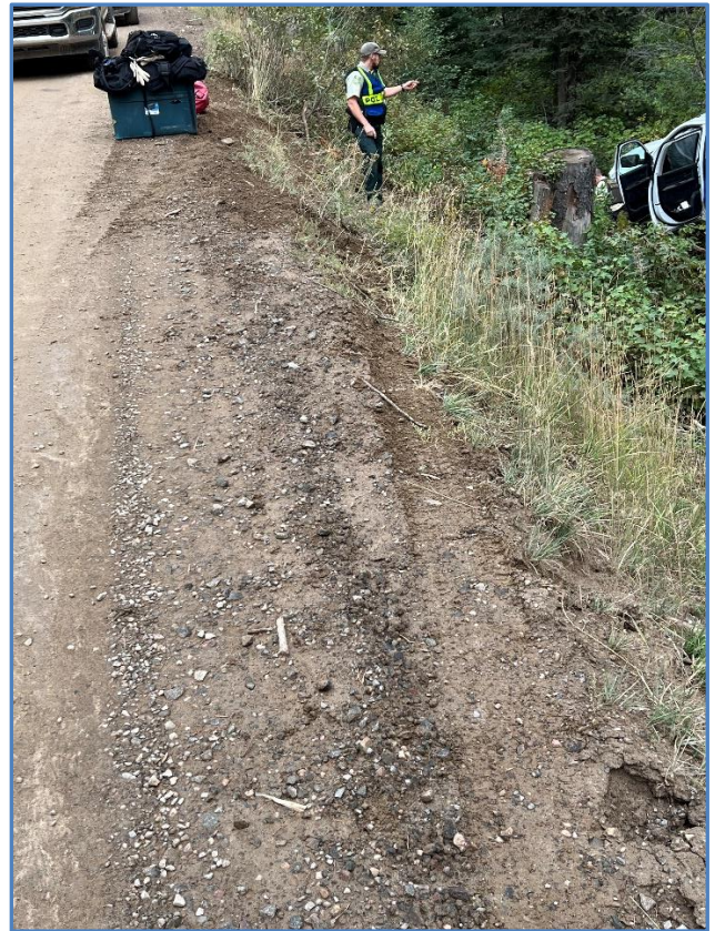
Tire tracks are visible where the truck's wheels were pulled off the shoulder into the “soft” dirt—and the vehicle rolled down the embankment.
